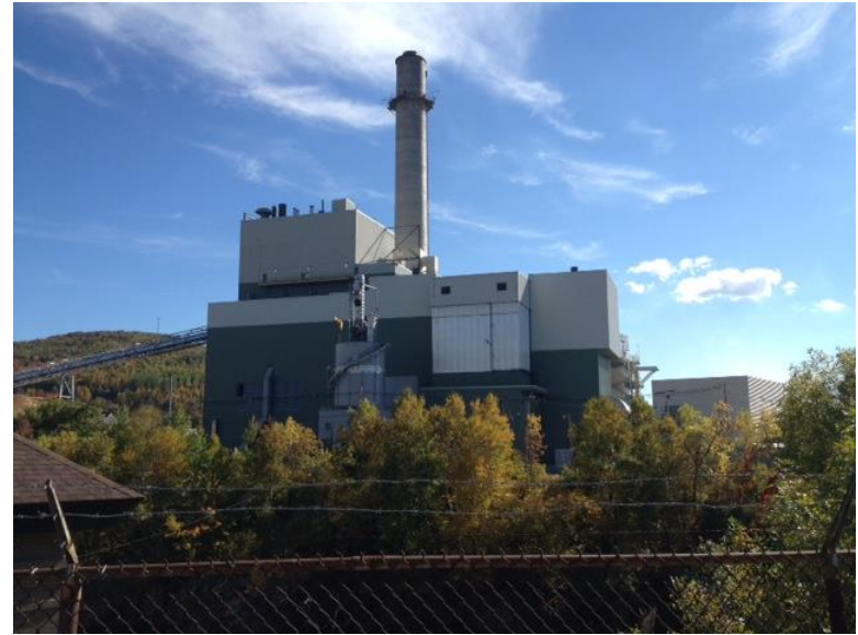
Frasier Pulp Mill in Berlin. Photo Credit: North Country Council
