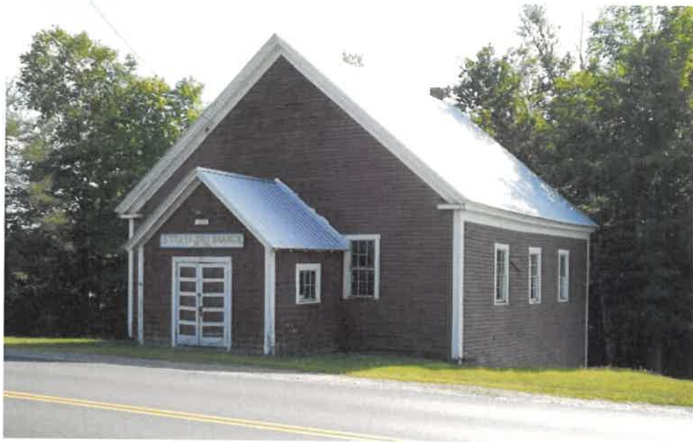
East Elevation of Grange
